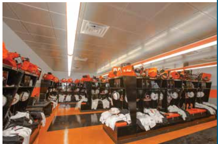
ROCKFON provided the schools' ceiling suspension systems, open plenum metal ceiling system, curved and straight specialty metal ceiling panels and perimeter trim.
