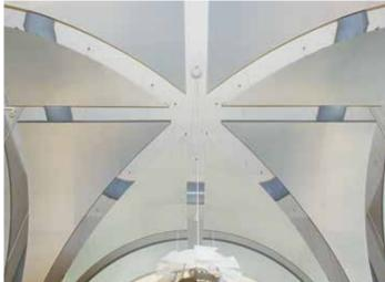
According to the installer, the particular challenge for this project was making sure everything lined up. It looks simple and seamless, but the design involved precision installation. Each individual ceiling cloud is free floating and the spacing between each sculpture piece had to be exact.
