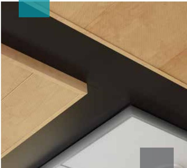
Accommodating the lights and air diffusers, the custom-sized Planostile planks were finished in both black and in Satin Silver. The Satin Silver was matched with Rockfon Infinity perimeter trim for a clean, smooth edge. Beyond the numerous sizes of factory-cut panels, the large columns in the main lobby also proved challenging.
