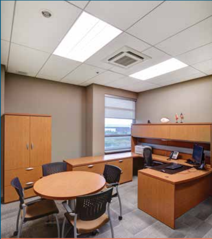
In nearly all of the private, closed offices, ROCKFON Sonar dB panels were installed to provide high sound absorption and minimize sound transfer between adjacent spaces to enhance privacy.
