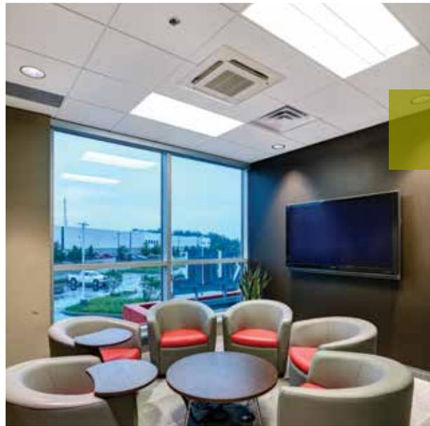
In nearly all of the private, closed offices, Rockfon Sonar dB 2-by-4-foot panels with a square tegular narrow edge are installed in Chicago Metallic 4600 Ultraline 9/16-inch suspension system. Sonar dB offers an elegant, lightly textured surface, high sound absorption and minimizes sound transfer between adjacent spaces to enhance privacy.
