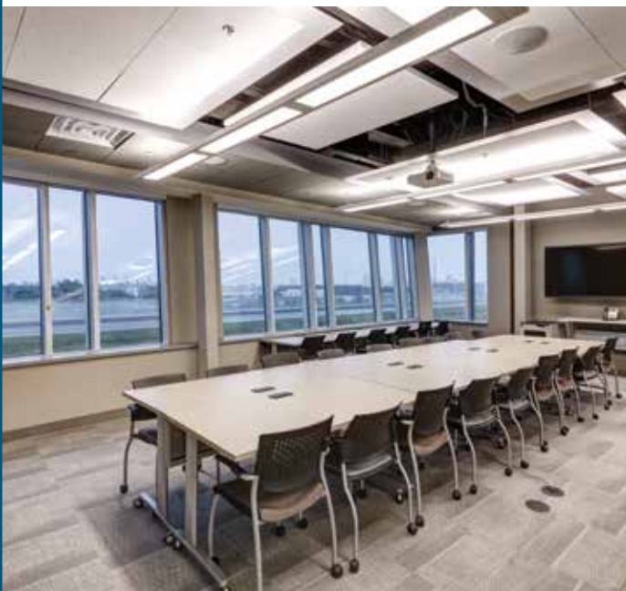
In the large group training room, ROCKFON Island products and Alaska ceiling tiles form clouds to deliver the acoustic performance essential to training.
