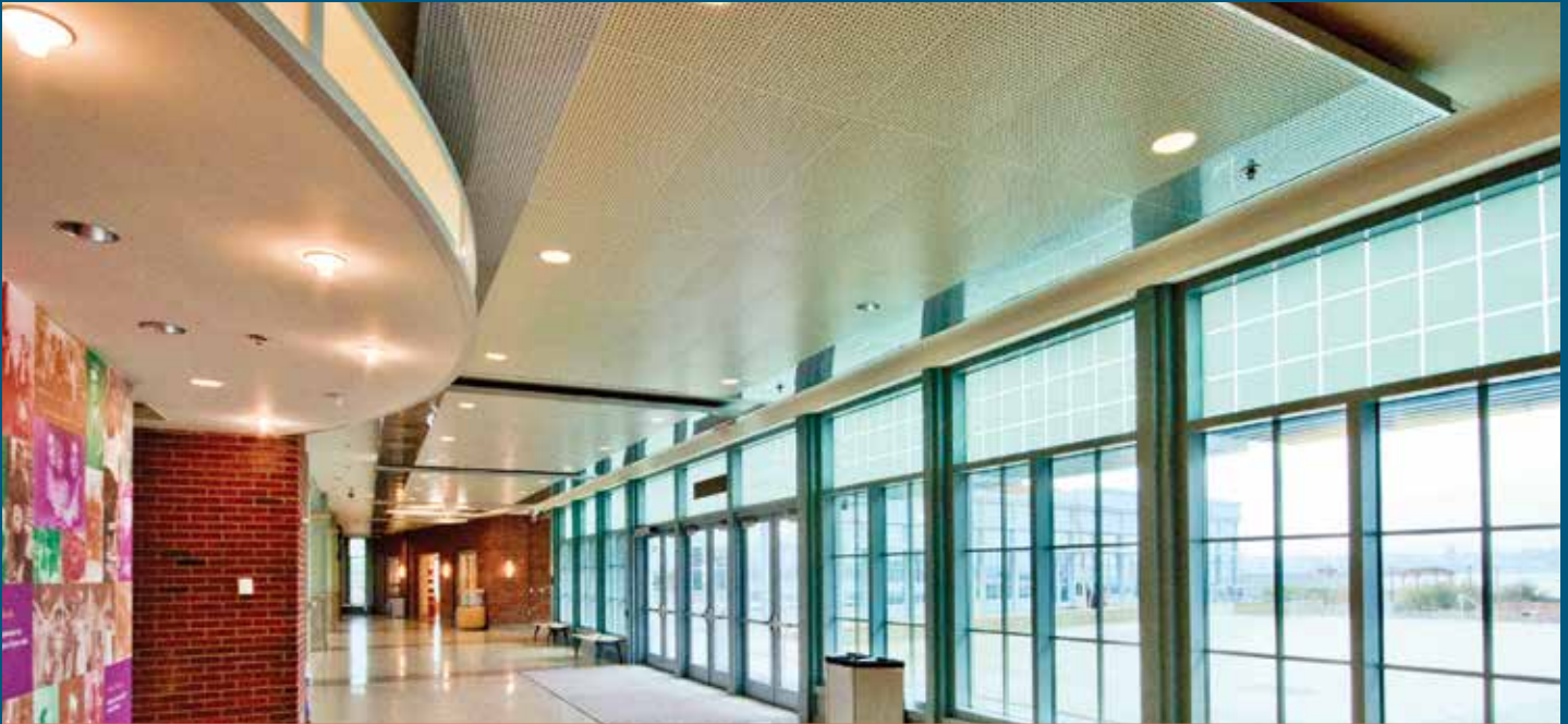
Floating clouds of Rockfon Planostile Snap-in metal panels guide the eye and help minimize the noise of foot traffic.
