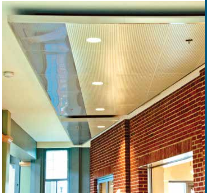
Various panel sizes and shapes were customized to align precisely with other architectural features of the building.
