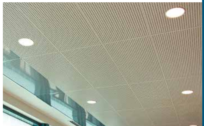
Rockfon's Planostile® Snap-in metal ceiling panels with Rockfon Infinity™ Perimeter Trim and Chicago Metallic's Seismic 1200 suspension system were used extensively throughout the NC History Center to create the floating clouds.
