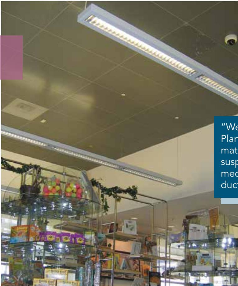
“We chose [Rockfon’s] Snap-in Planostile ceiling system for its materiality, as we needed a suspended ceiling to cover the mechanical systems such as duct work and pipes.”
