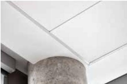
Rockfon's stone wool ceiling panels are made from basalt rock and contain up to 42 percent recycled material to support ESCB's LEED Gold criteria. Stone wool ceiling panels also are lightweight and cut easily to accommodate the facility's columns, light fixtures and sprinklers.
